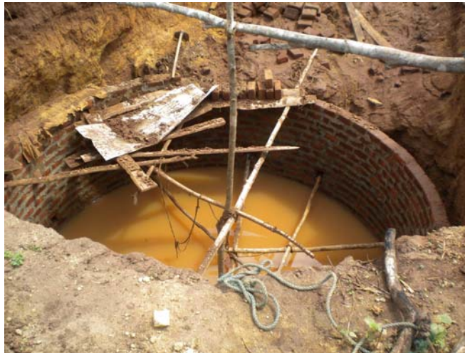
put in aanbouw in Mahairikewa
